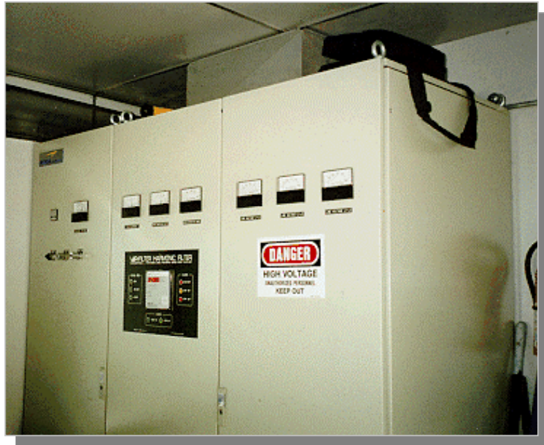
Example of a harmonics filtering system installed by VAR+Technologies at Keystone
