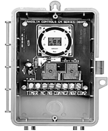
Grasslin timer installed on Snowmass Mountain
